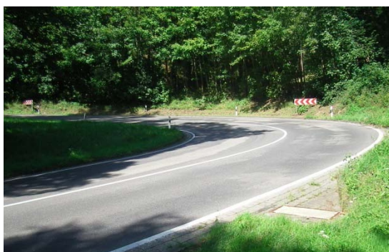
Figure 2: Observation site at a curve (Linz / Germany) /BAST/
