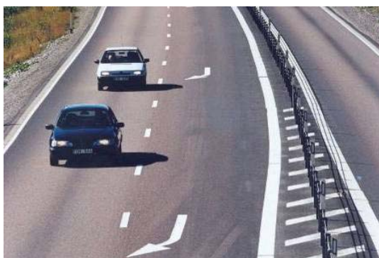
Figure 3. Road with a wire rope median guard rail to avoid head-on collisions.
