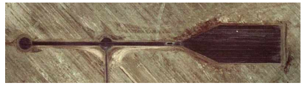
Figure A5. Dynamic Research Inc. Skidpad, 800 ft. x 300 ft., Shafter, CA
