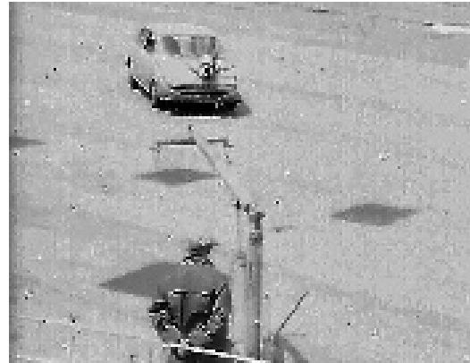
Figure 4. Demonstration of BL 1300 Pedestrian Safety car with catcher, TRL, 1974 ( abergraffic )
