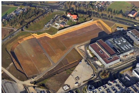
figure 6: Start of construction, April 2014
