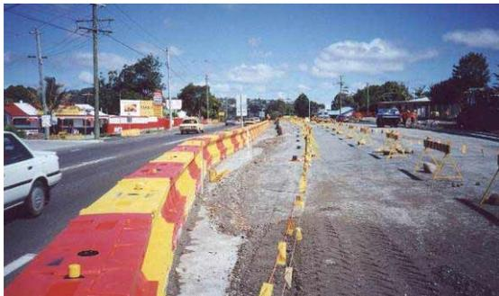
**Figure 6 Waterfillable Roadliner barriers tested and certified to AS/NZS 3845.**
