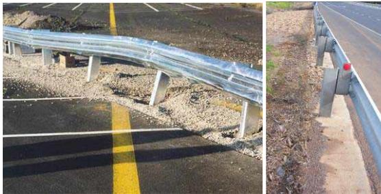
**Figure 11 Guard rail barriers. Left: posts move in soil. Right: post set in concrete.**
