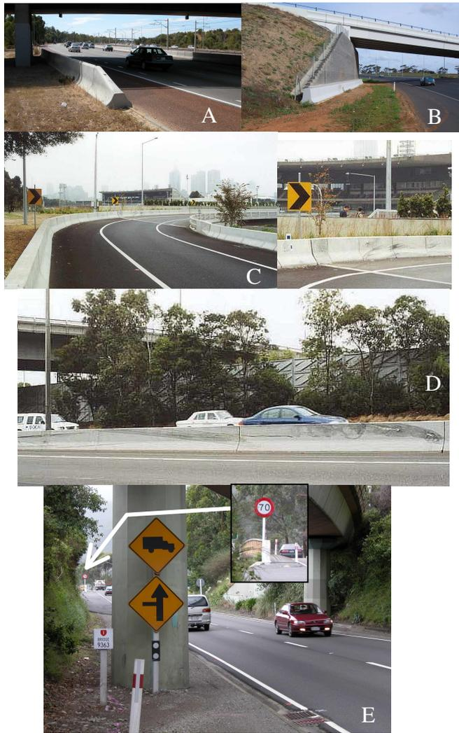
**Figure 21 Real world lethal roadside hazards in Australia and New Zealand.**
